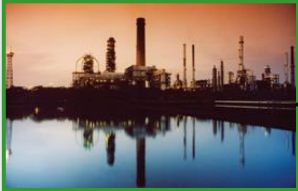
MATHURA REFINERY 8 MMTPA
